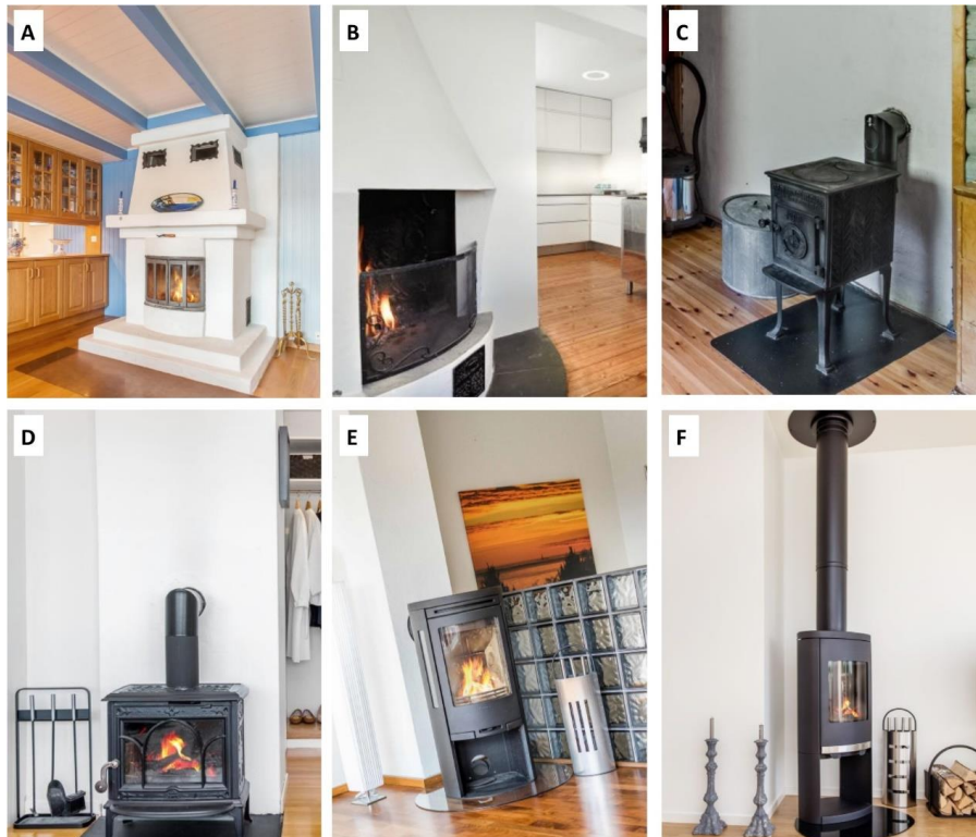
Figure 1: RWC appliances commonly used in Norway. A and B: Fireplaces. C and D: old stoves produced before 1998. E and F: new stoves produced after 1998. (Photos are from finn.no)
