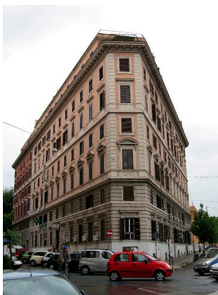
Figure 1. Soiling of a building facade and windows in Rome, Italy.
