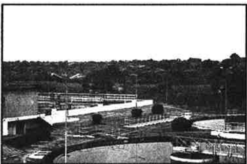
Water treatment plant
