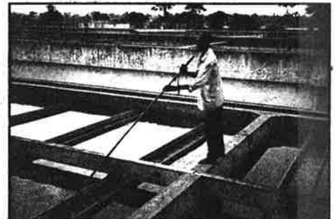
Water treatment plant maintenance
