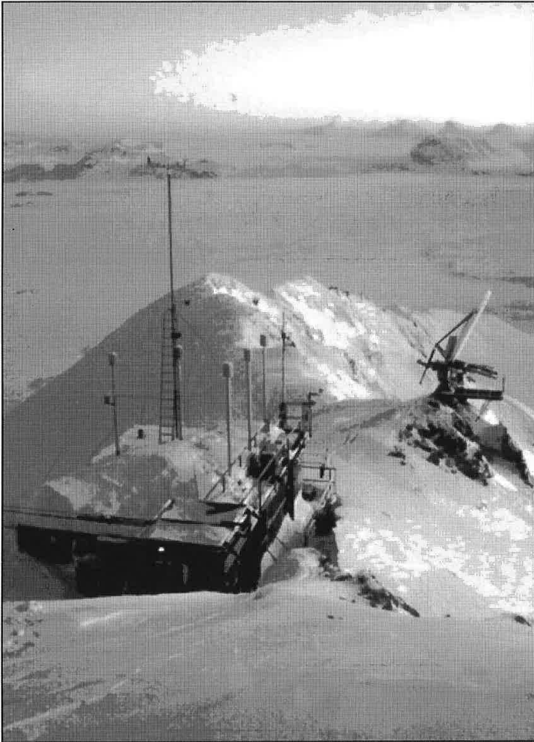
Figure 6. The Zeppelin mountain station.
