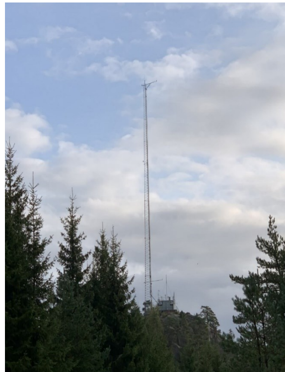
Figure 59: Birkenes Observatory with the new 75 m mast installed August-September 2020 to comply with the ICOS requirements.
