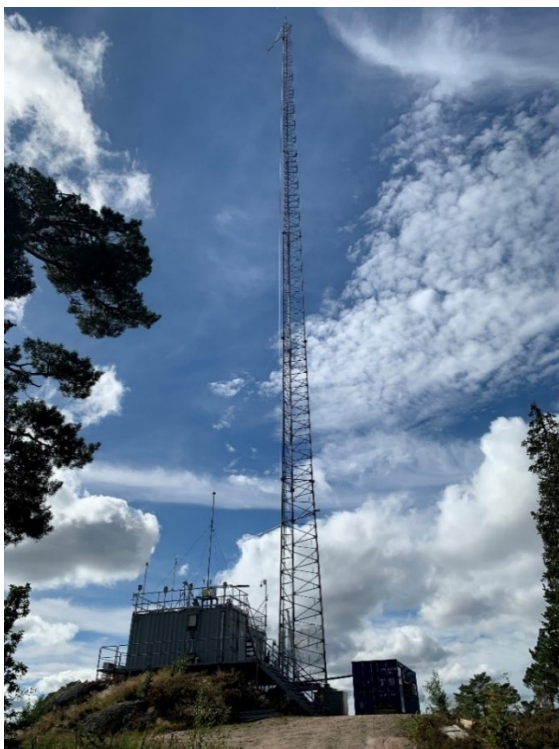
Figure 59: Birkenes Observatory with the new 75 m mast installed August-September 2020 to comply with the ICOS requirements.
