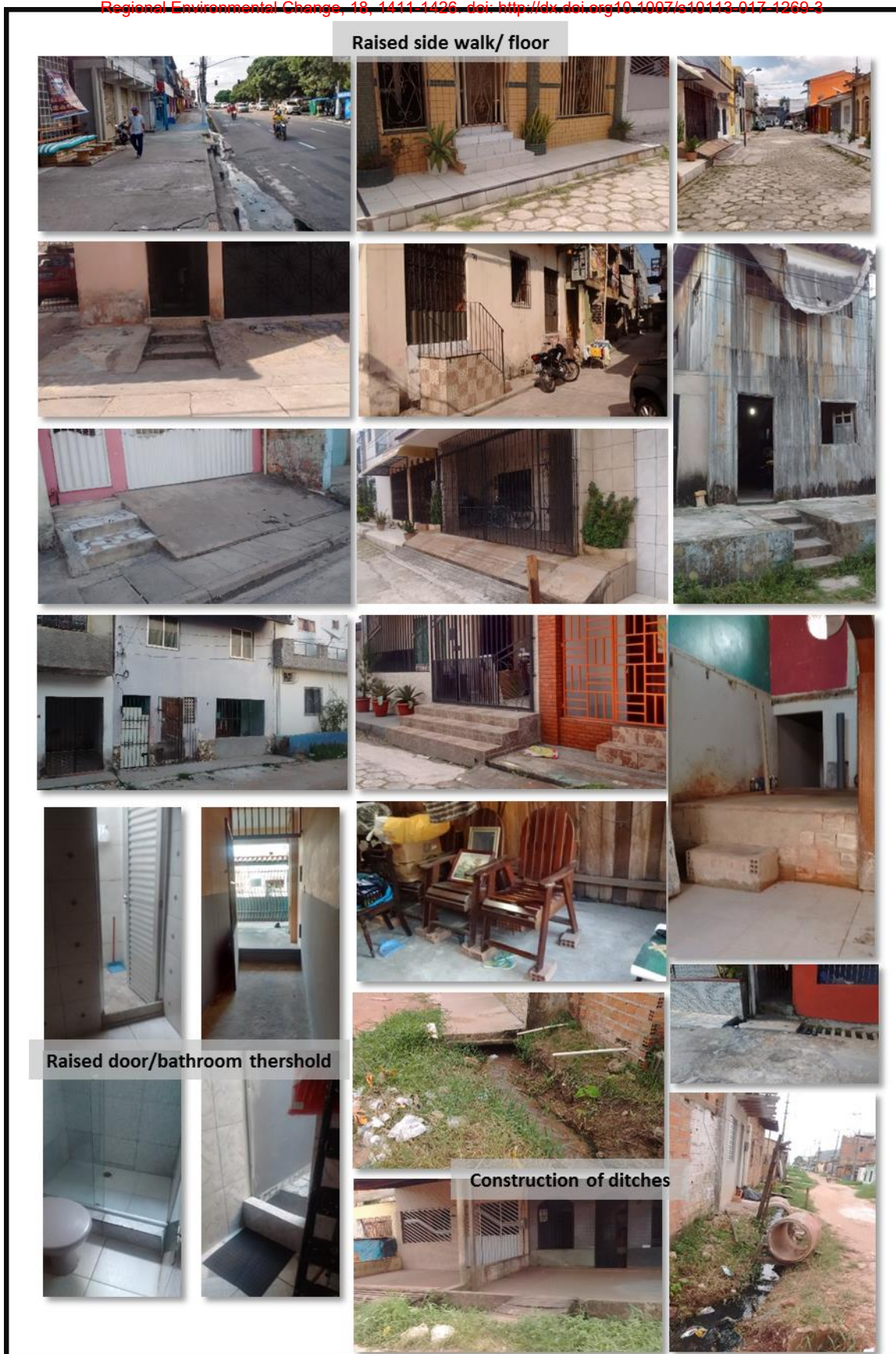
Figure 5. Examples specific adaptations to flood risk at the household and community levels in the city of Belém.
