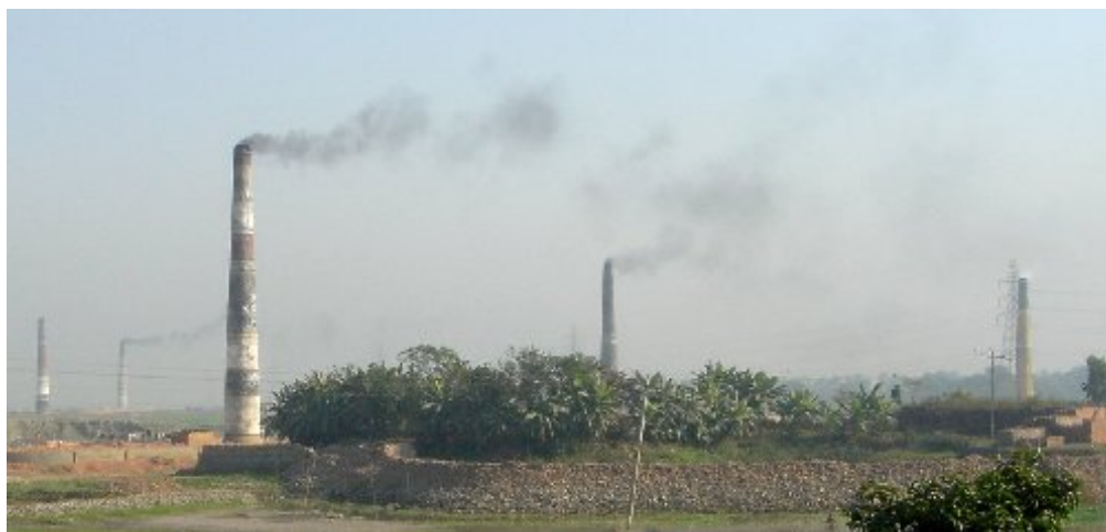
Figure 9: The brick kiln area around Gabtali consists of 108 stacks each between 40 and 50 m high.
