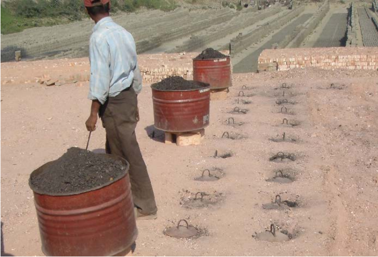
Figure 10: A Hoffman type furnace where coal is fed into the kiln through holes from above.
