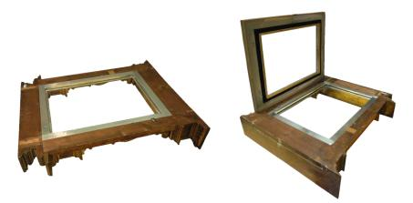
Back of frame; original wood sealed with aluminium tape (left); microclimate frame hinged onto original frame (right)
